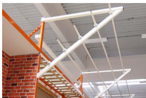
Projecting elements, e.g., for hoists (top right) and ventilators (right with moving holders)
