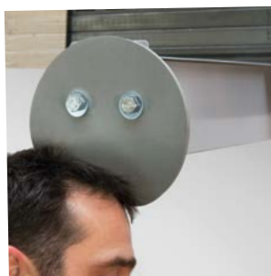
Rubber head protection for cantilevers at head height
