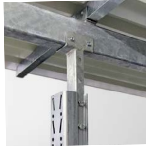
Connection to the shelving system; long and short holders result in the roof pitch
